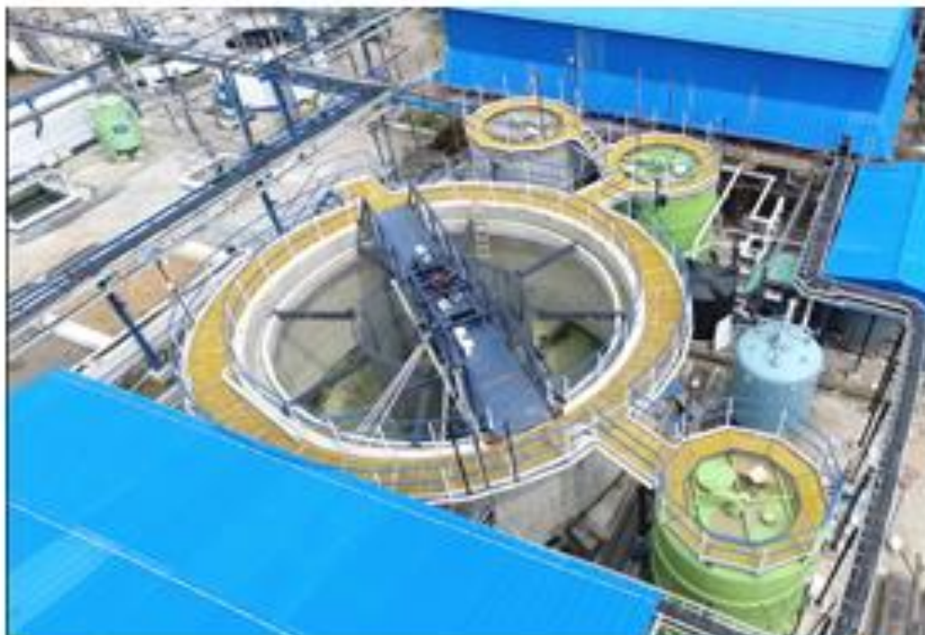
Effluent Recycling Plant Overview (40 m 3 /Hr)
